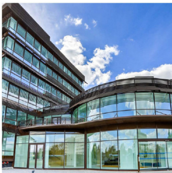
HELIS BUILDING Vélizy, France
