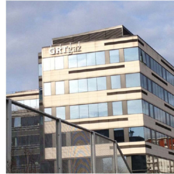
GRT GAZ Bois Colombes, France
