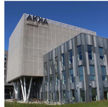
AKKA Montigny-le-Bretonneux, France
